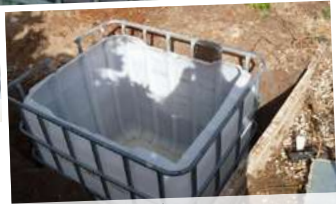
Sump tank finally in it's hole
