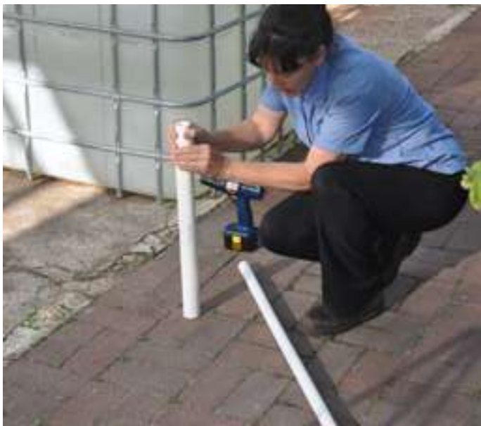
Making the standpipe which controls the water level in the growbed
