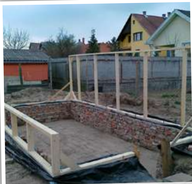
Greenhouse walls being constructed
