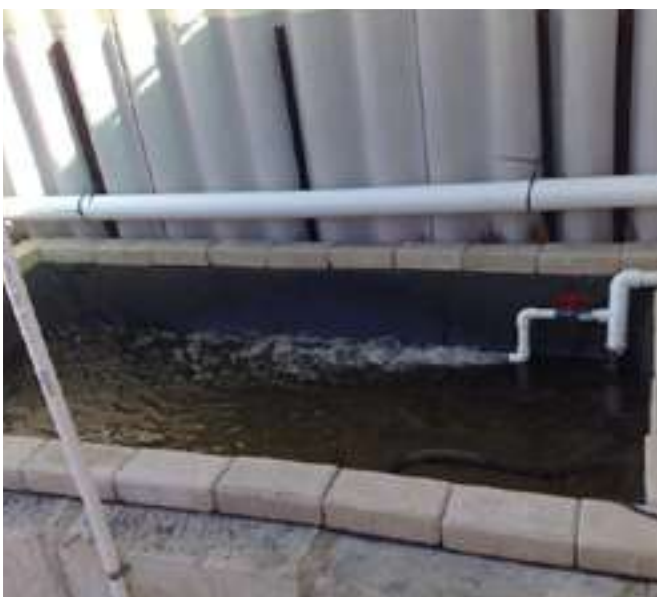
The main sump tank what contains the pump; Sumps all set up, stands partially buried to a better height
