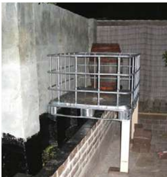
IBC growbed supported at the back with bricks and at the front steel legs were bolted on to provide the support
