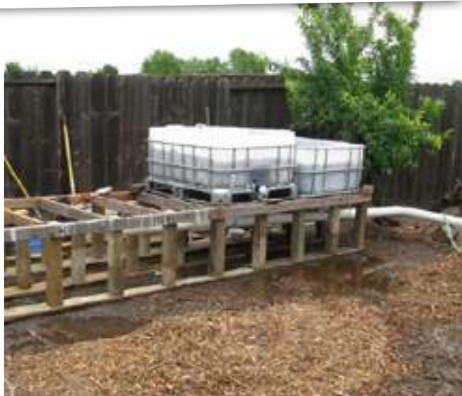
Solid timber stands are required to support the weight of growbeds
