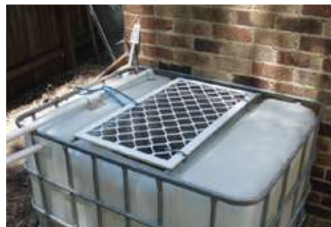
Security screen stops unwanted visitors and debris entering the container and can be opened to gain access for fish harvest
