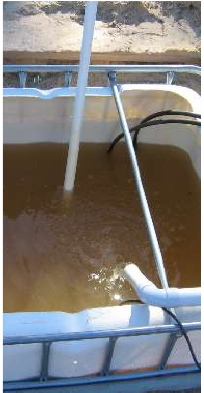
Sump tank buried and supported in ground
