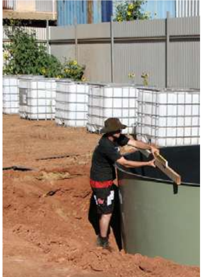
Positioning the enormous fish tanks
