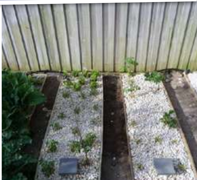
Growbeds installed at ground level and all drain pipes buried. Irrigation line runs along the fence behind
