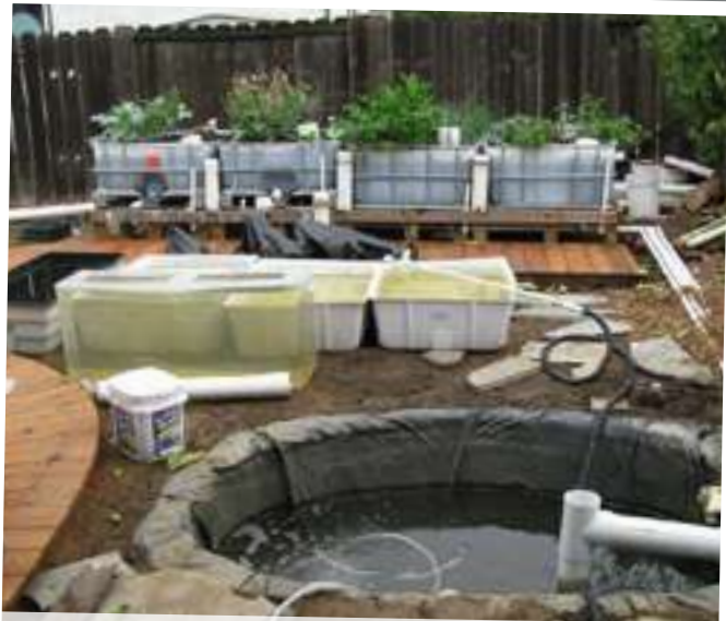
Renovation in progress
