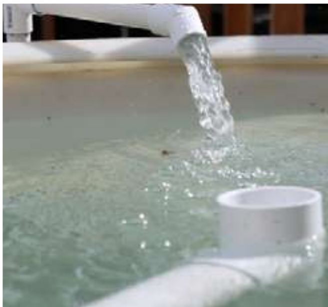
Inflow from the sump into the fish tank
