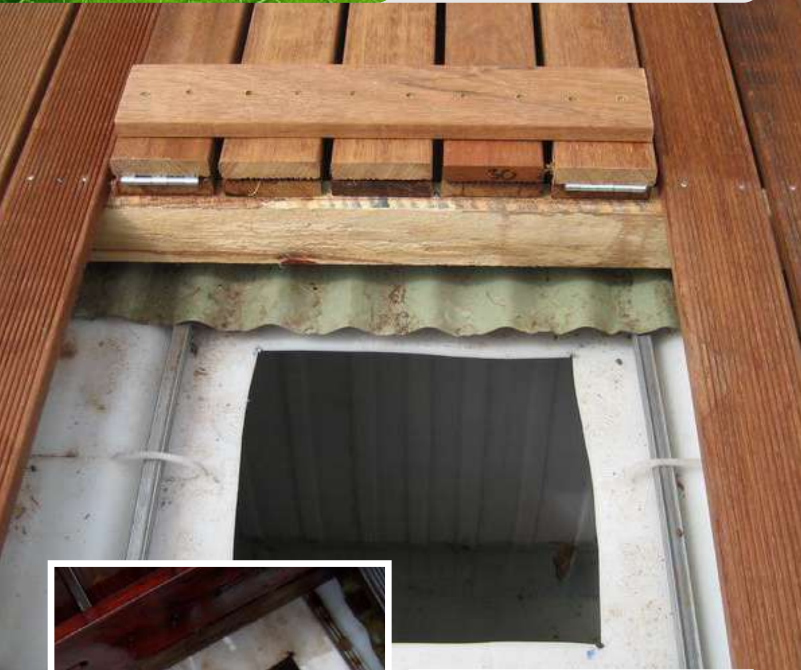
Decking is hinged and can be accessed when required
