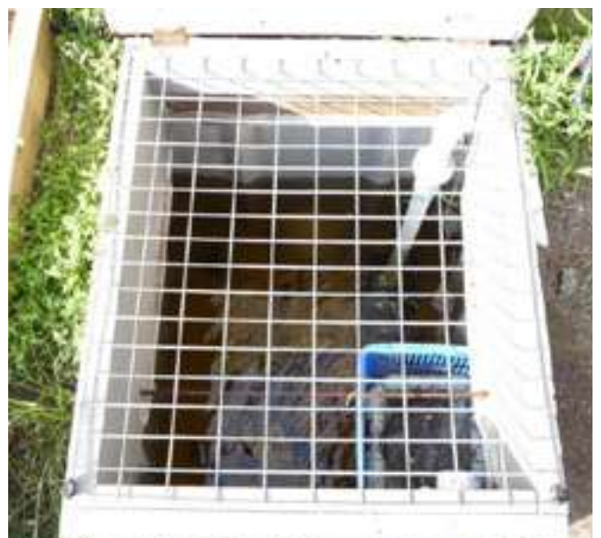
Buried IBC with childproof cover
