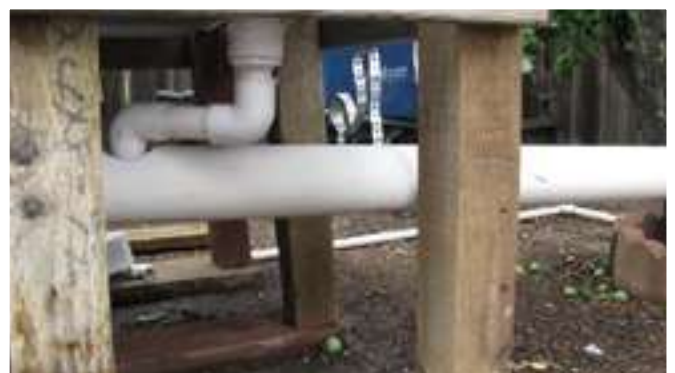
Drain from growbed to 4' drainage pipe back to pond
