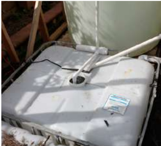
All the growbeds drain into the sump tank before the water is pumped back into the fish tank
