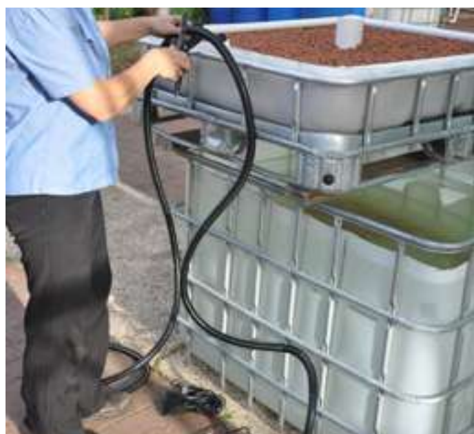
Measure and cut the flexible anti kink pipe
