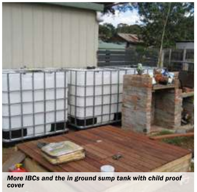
Decking is hinged and can be accessed when required
