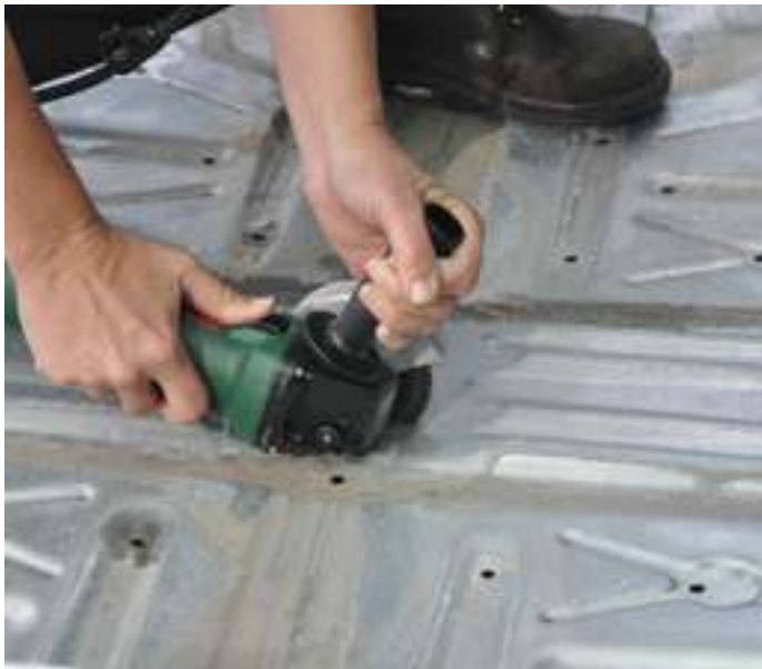
Cut the hole in the steel base large enough for the drain fittings
