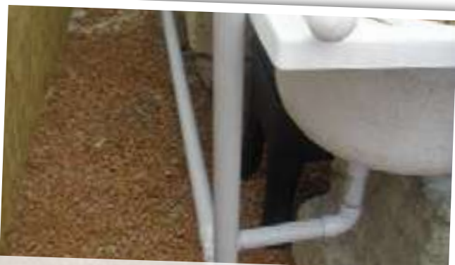
The drain pipe has a breather; Gravel growbeds are very neatly laid out
