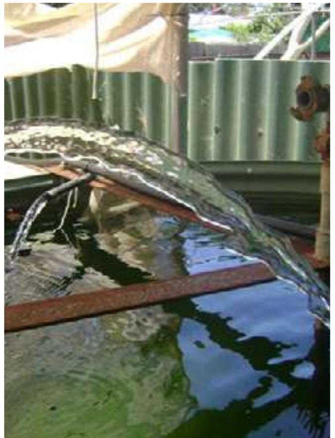
3000 litre rain water tank added to the system
