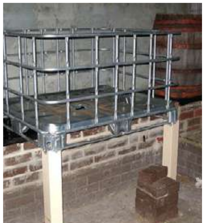
The metal base for the IBC is just deep enough that it can fit a 90 degree outflow pipe
