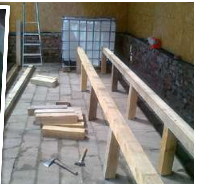
Heavy duty beams to support the growbed
