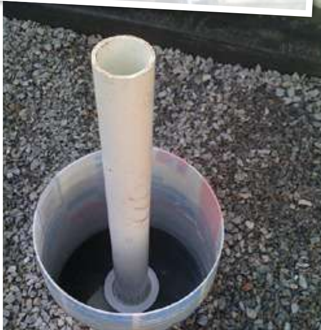
Simple standpipe with surround acting as a media guard
