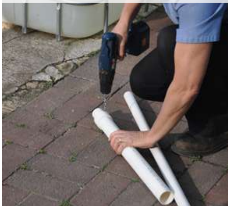
Drill 6mm holes in the standpipe and the irrigation grid pipes
