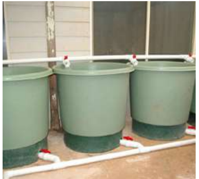
Irrigation and drain lines set out
