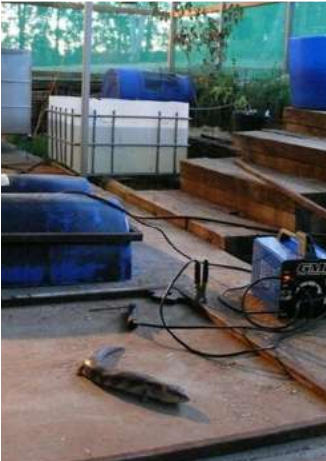
Framework for the barrels under construction
