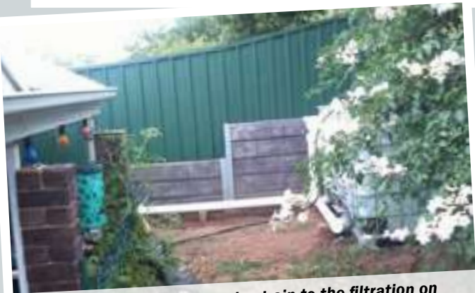
IBC's on the right showing the drain to the filtration on the left
