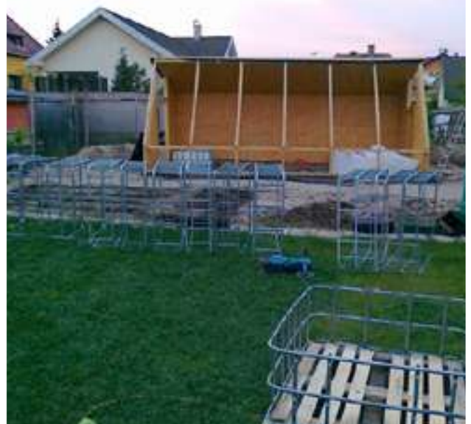
Growbed frames and one sump frame
