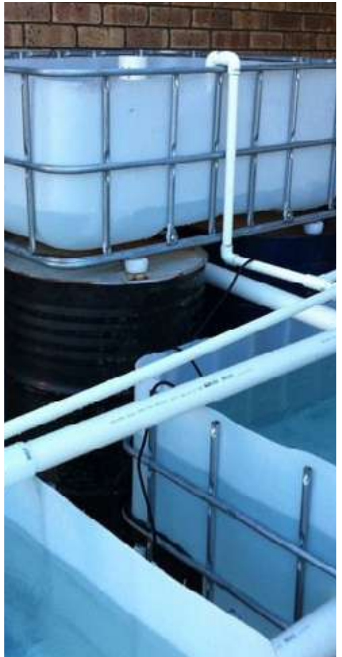
Pipes are checked for leaks
